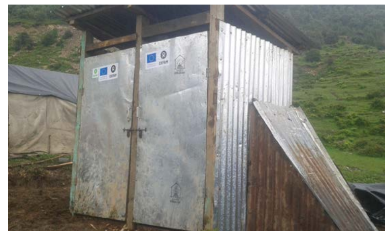
Figure 4 and 5: Direct disposal to a storage bin from a chute inside the cubicle (Oxfam-Nepal, 2015)
