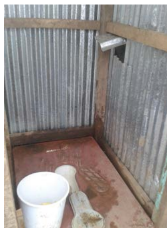
Figure 4 and 5: Direct disposal to a storage bin from a chute inside the cubicle (Oxfam-Nepal, 2015)
