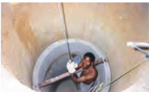
Well construction. Photo: WASH visual aids library
