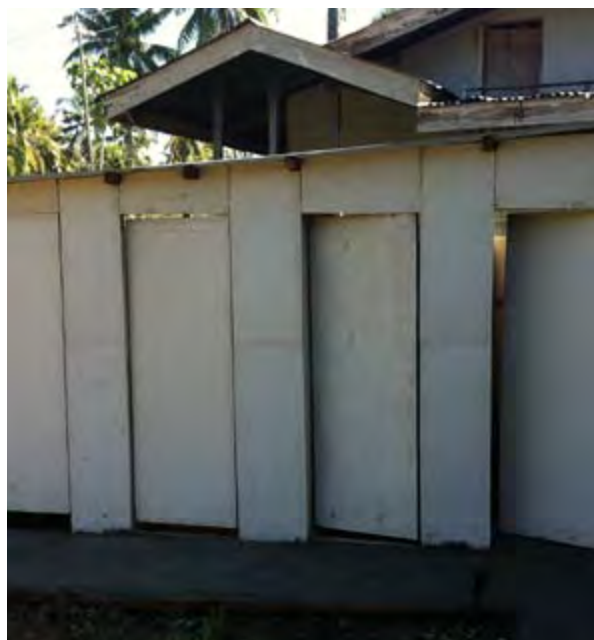
Figure 16 Latrines constructed with plywood/Photo by Kate Davis
