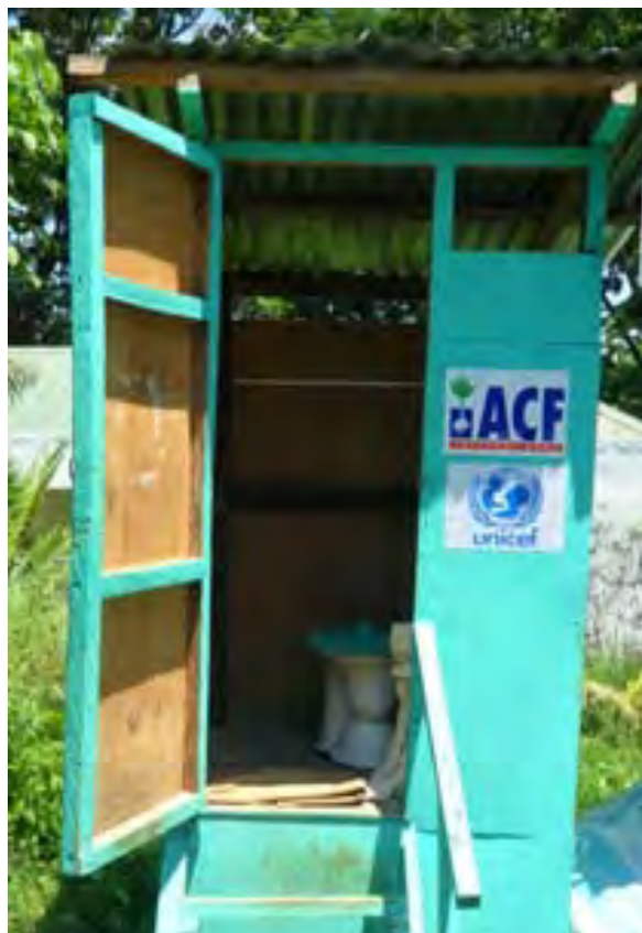
Figure 17 Recycled WAND EcoSan/Photo by Kitty Tiukinhoy
