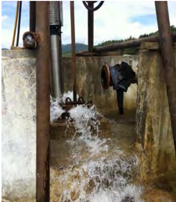
Figure 10. Iligan well production cleaning in Iligan/Photo by Kate Davis
